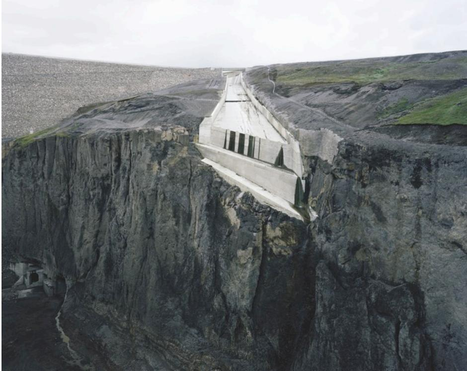
Concrete spillway chute, Kárahnjúkar dam, 2010
